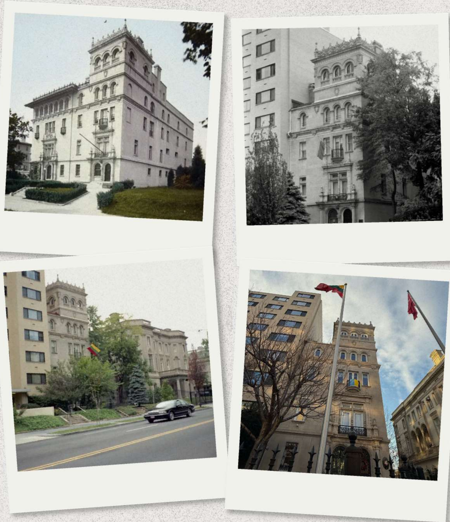
Photos: Lithuanian Embassy Throughout Years 1st photo: The original duplex of the Embassy of Lithuania, until the building at 2620 Sixteenth Street was torn down in 1965 and replaced with an apartment complex. Photo courtesy of the Library of Congress.
